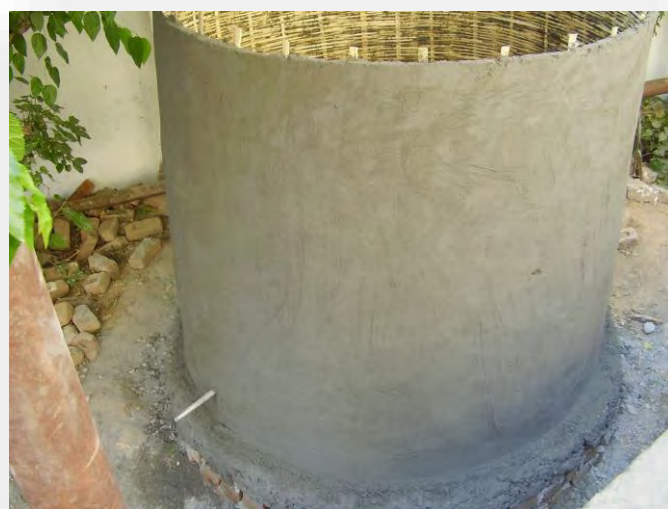
Fig 5.2.6 Bamboo based rain water storage tank
