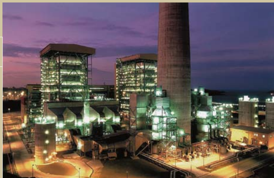
Sual 1,200 MW coal-fired power plant
