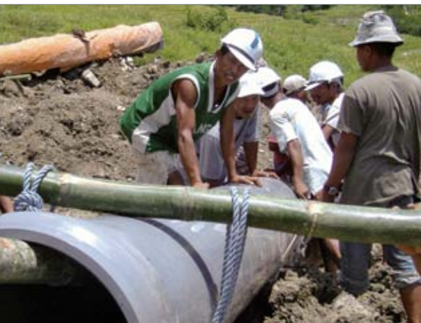
Installing the penstock pipe sections
