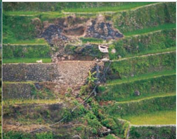
The deterioration of the rice terrace walls has a cascading effect.
