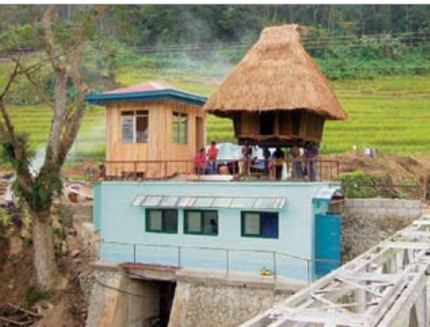
Ambangal powerhouse composed of a power-generating equipment room, an operators room and accommodation in a traditional house
