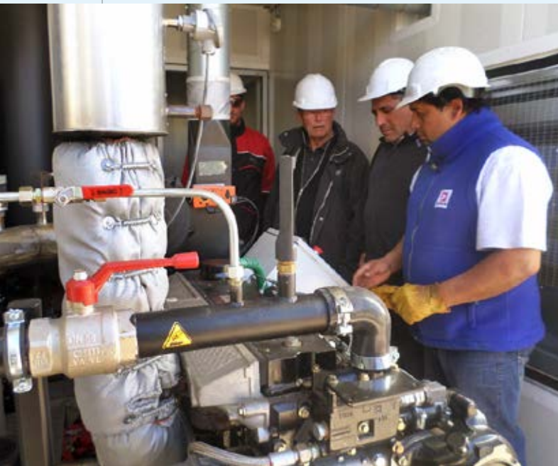
EPEN operators receive training on the new wind generation electric system
