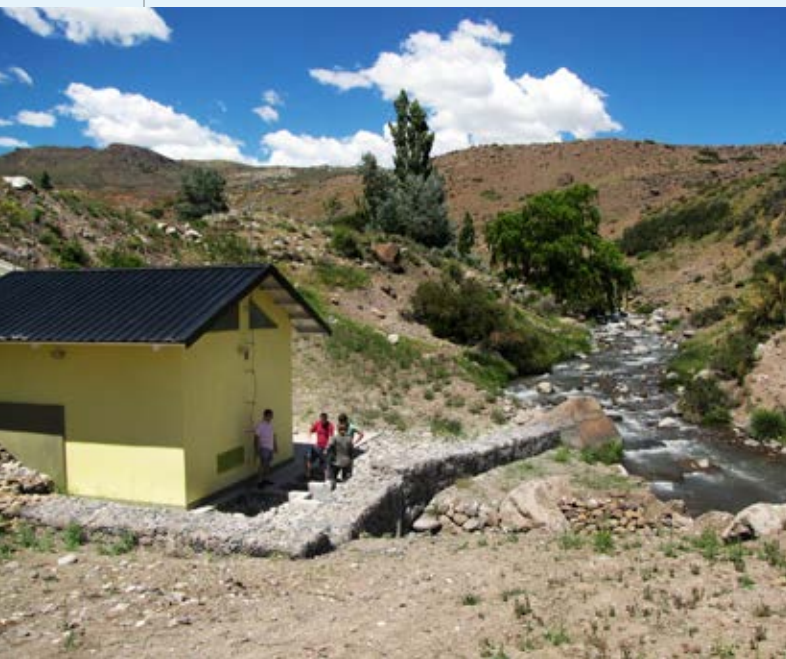
The new Cochico Mini-Hydro Power Plant and its power house
