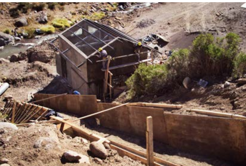
Cochico's plant power house under construction
