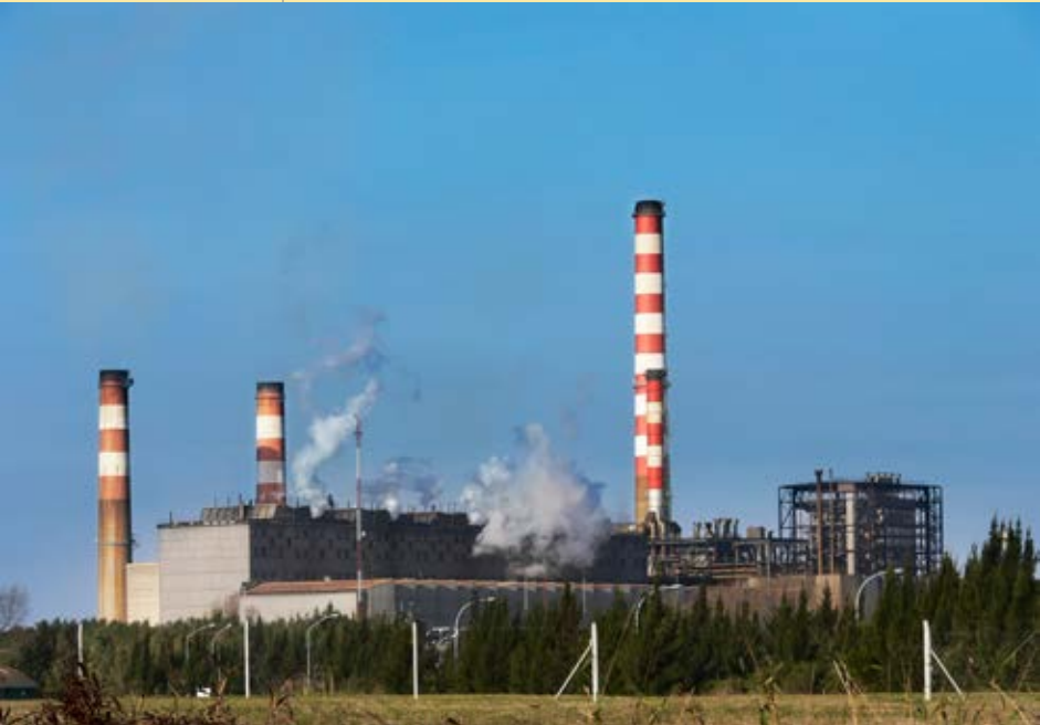
Thermal power plant near Buenos Aires, Argentina
