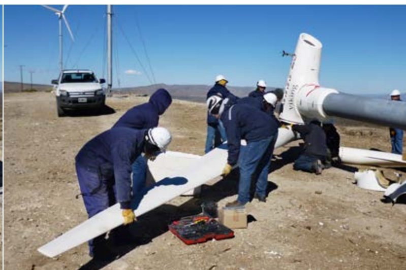
Workers assembling one of the wind turbines on site
