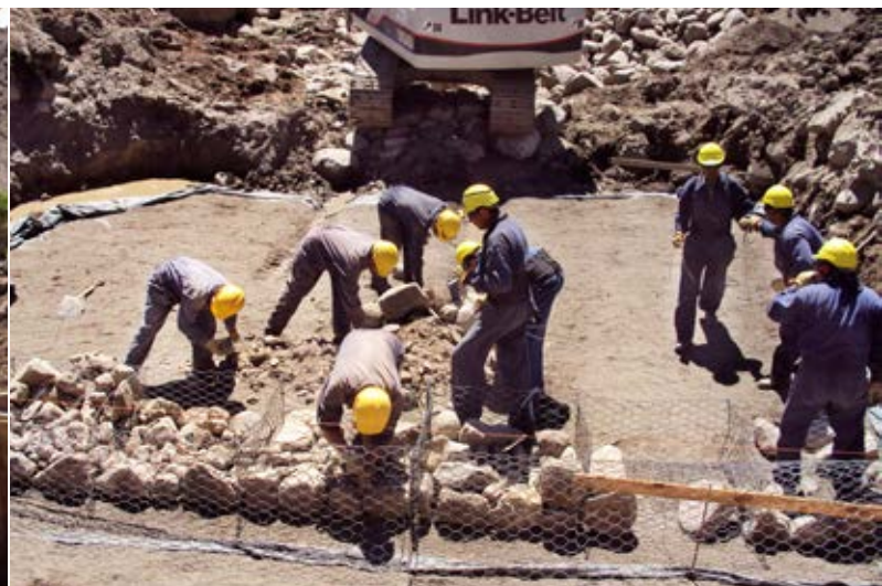
Works under way for the power plant's intake structure
