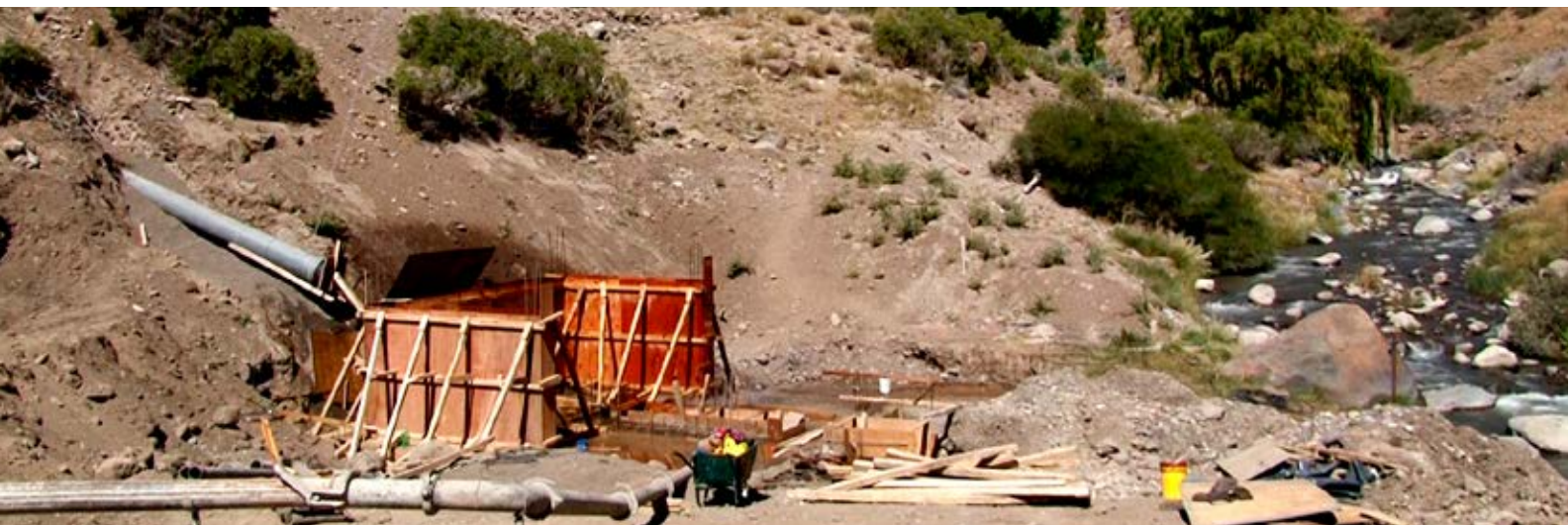
Cochico mini-hydropower plant under construction
