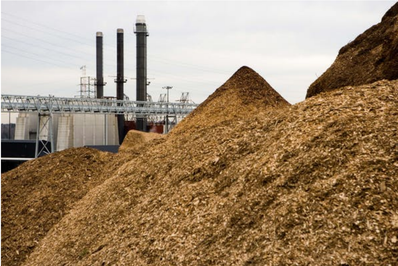
Wood yard, Schiller Station, Portsmouth, New Hampshire. One boiler at the four-unit plant was converted to wood in 2006 and has consumed more than five million tons of wood fuel. PSNH/Flickr, CC BY-ND
