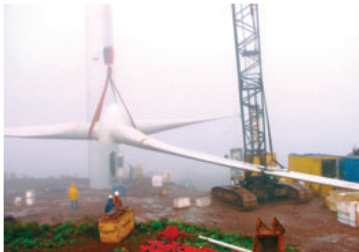
Wind turbine blades being lifted by special cranes
