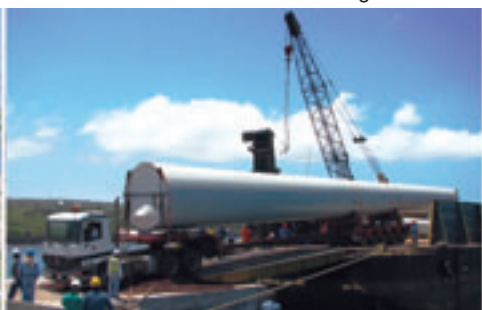
Off loading wind tower
