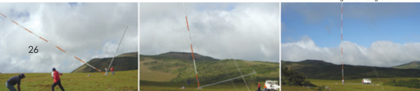
Wind measuring tower being lifted
