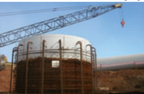
Tower anchoring rings
