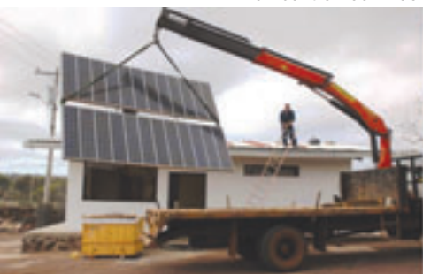
6 kW solar panels installed on control room roof
