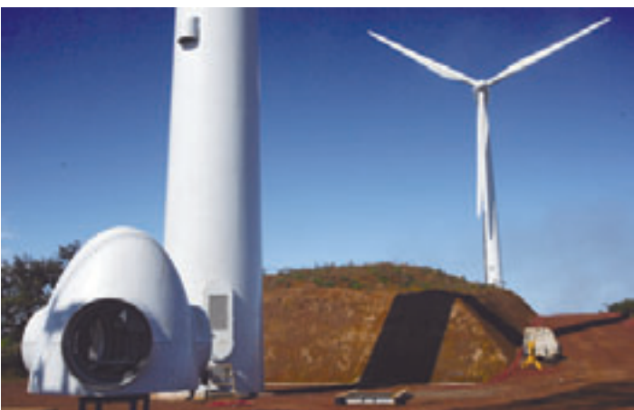
Wind turbine during installation process
