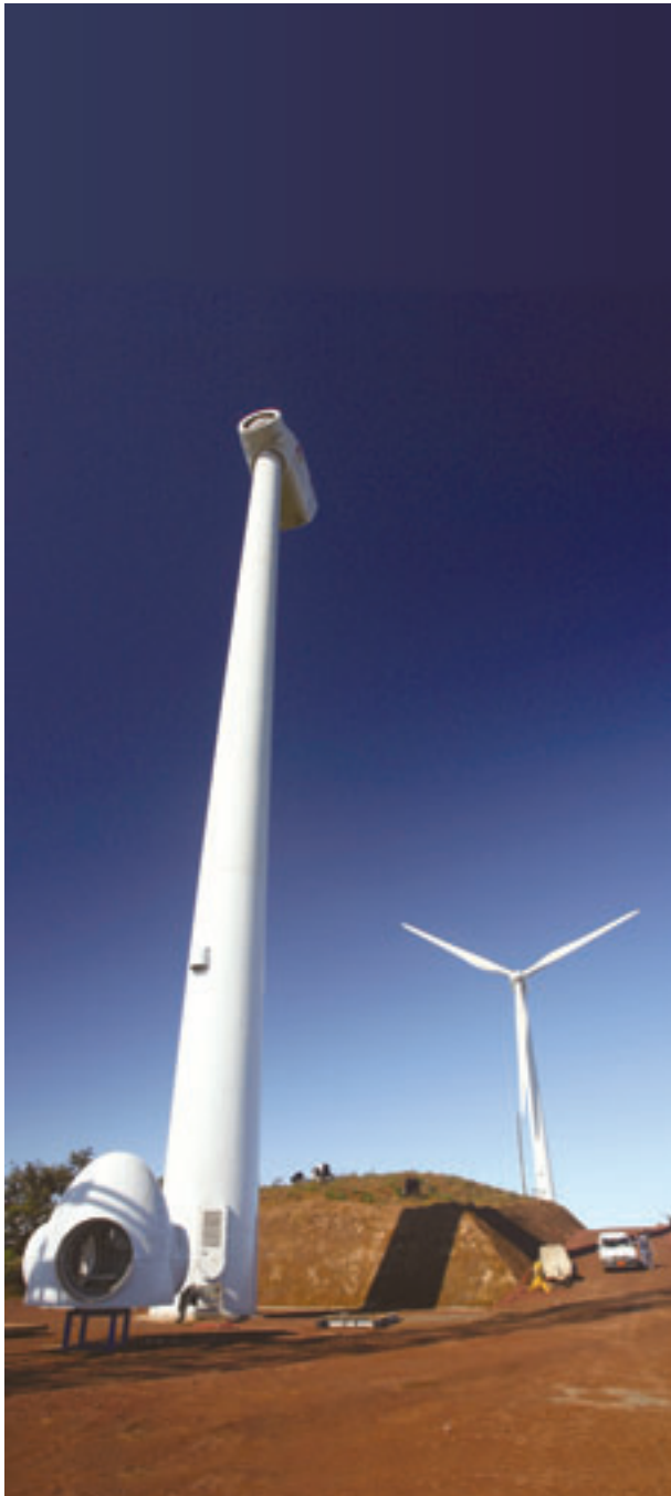
Hub ready to be lifted at wind turbine No. 2
