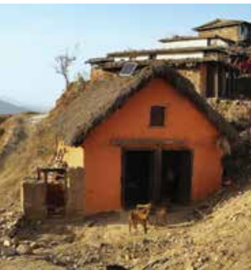
Example of an off-grid solar home system in rural Nepal
