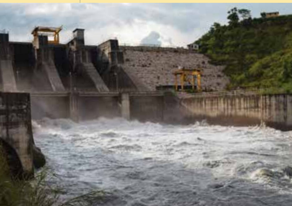
The Marsyangdi Hydropower Plant in Nepal
