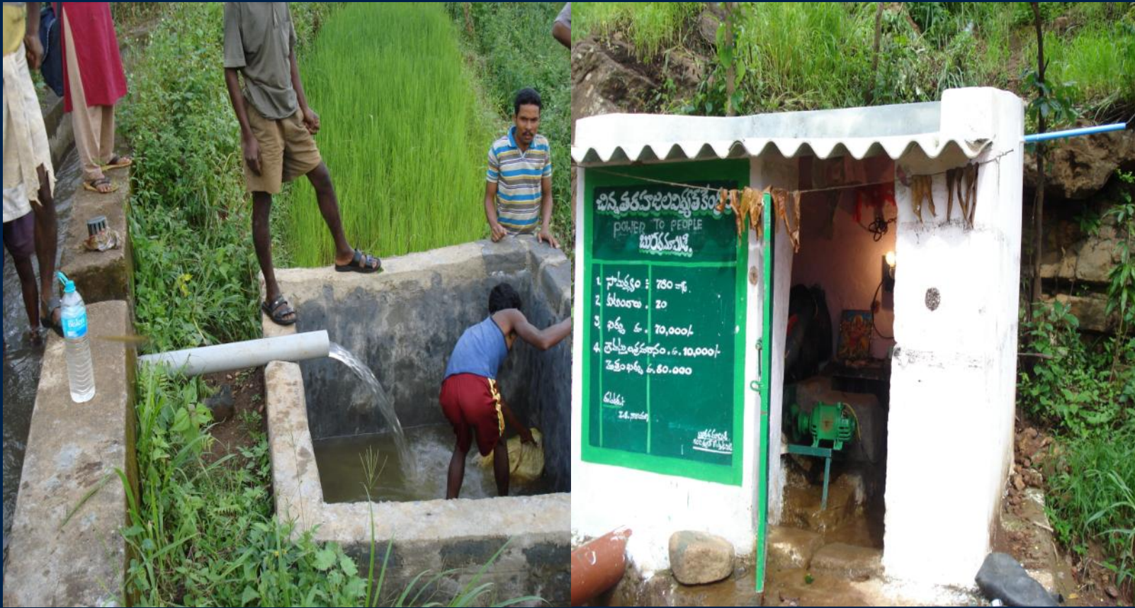
A 'Nano' Hydro (less than 1 KW) at work, Burdhamamidi, Peddakodapalli Panchayat, Peddabayulu Mandal, Visakhapatnam District, Andhra Pradesh
