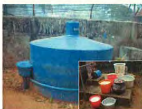
Fig. 8 A decentralised anaerobic digestion in Kerala, India
