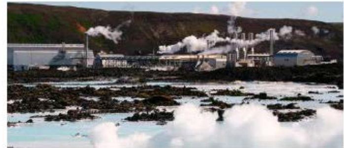
Svartsengi (Blue Lagoon) CHP plant: 76 MW e. 100 MW th. Utility: HS-Orka. In operation since 1977. Wells 24.
