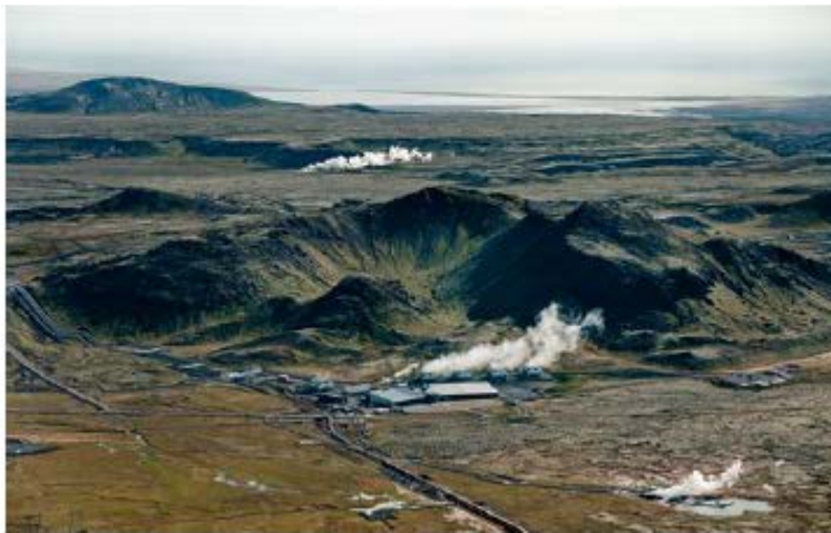
Hellisheiði CHP plant: 303 MW e. 133 MW th. Future plan +267 MW th. Utility: Orkuveita Reykjavíkur. In operation since 2006. Wells 71. 5.10.2012
