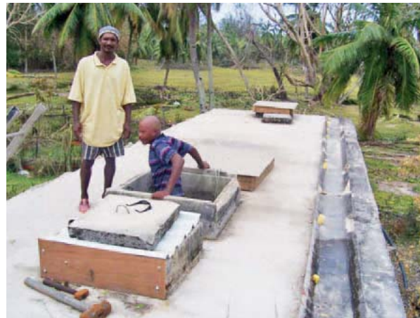
Figure 2: Concrete water storage tank, drained to create a shelter from intense cyclone Bondo | Source: DRDM, 2007
