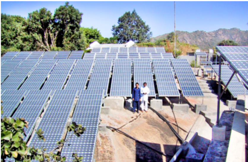
150 KW PV system with battery backup, Gyan Sarovar, Mt. Abu
