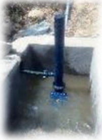
Hydraulic Ram Pump (Hydam)
