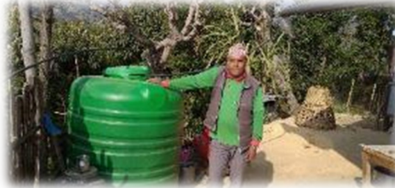
Rooftop Rainwater Harvesting
