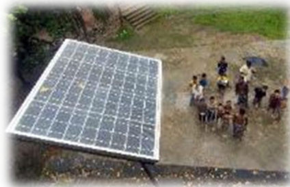
Solar Home System
