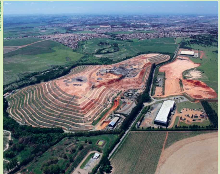
CGR Paulínia is a state-of-the-art disposal facility.
