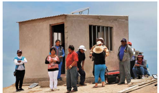
Rooftop mini solar lighting systems have been installed along the coast to improve the security of the fishermen at night.
