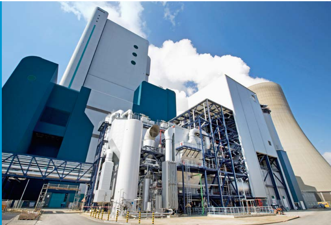
BoA 2&3, a lignite-fired power station with optimised plant engineering, operates at an efficiency rate of 43% in Neurath, Germany (RWE).
