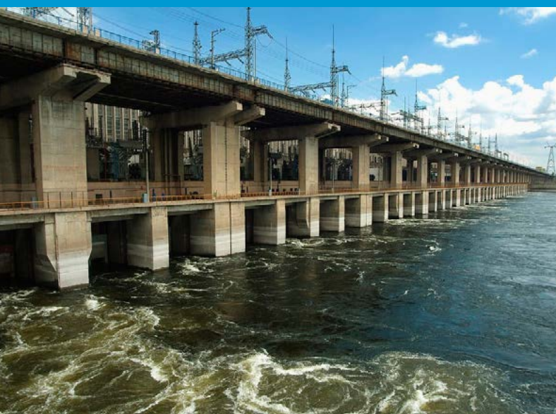
The Volzhskaya Hydropower Plant is the largest European hydropower plant with an installed capacity of 2,639 MW and 23 hydro units of various capacities. It is the last downstream power plant of the Volga River in Russia (RusHydro).
