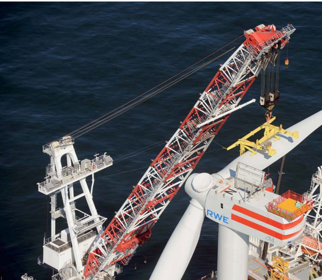
The Nordsee Ost offshore wind farm in Germany has an installed capacity of 295 MW and uses 48 multi-MW wind turbines in water depths of up to 25 metres (RWE).
