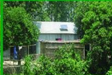
Installed Solar Home System at Khowamuri village
