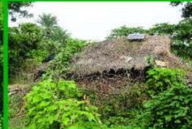
Solar Home system at remote village in Patuakhali
