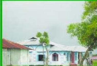
Solar Powered Mosque in cyclone-prone Patuakhali District
