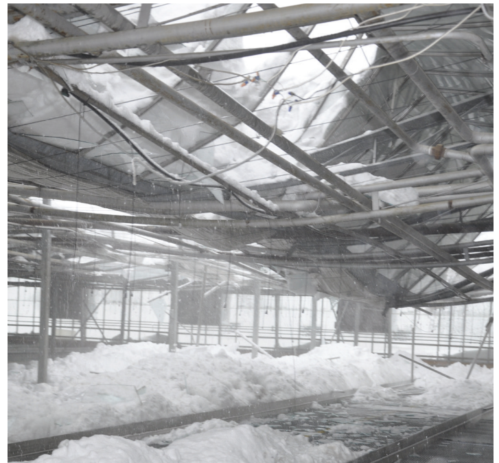
Collapsed Greenhouse in Western NY from the 2014 Snowstorm
