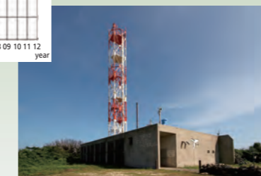
9 Hateruma Global Environmental Monitoring Station
